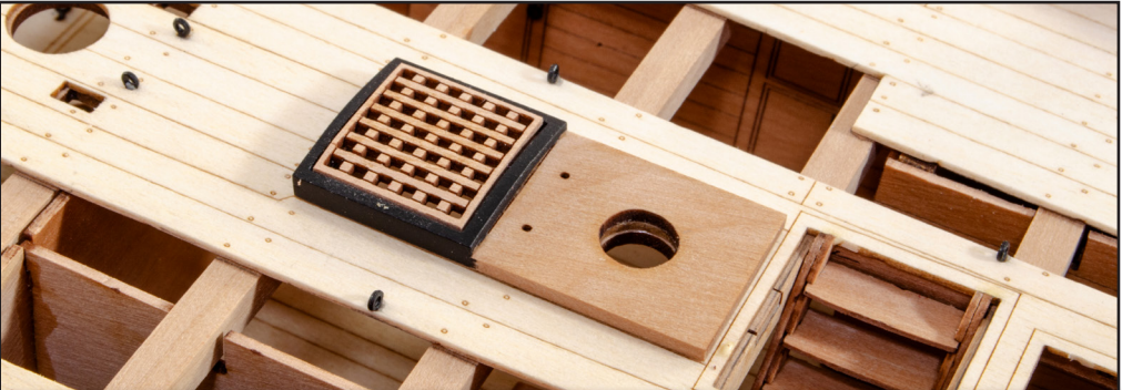
304. This last assembly can now be glued to the deck. Use a dowel to ensure that you get the mast hole properly aligned.
