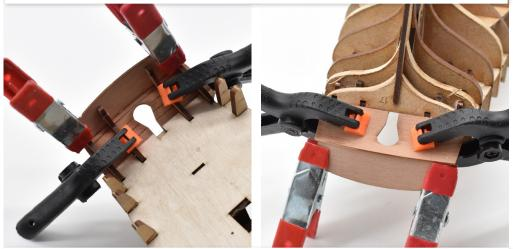
21. Using PVA wood glue, fix and clamp part 62 in place on the four stern frames, the engraved vertical lines liming up with each of the stern frames. Follow this buy gluing and clamping the inner stern transom (63). Leave for 24 hours to thoroughly cure.
