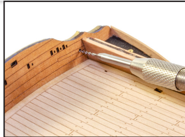
559. Use a 0.6/0.7mm drill and drill through the outermost holes in the transom until the holes breaks through the resin stern decoration. That is where the lanterns will later fit.
